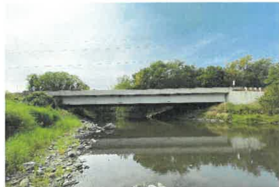
Bridge 86512 downstream of Bridge 86503
