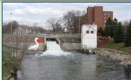
The deteriorating dam in Pelican Rapids, MN was modified into a Rock Arch Rapids winter 2022/2023. The ramp gradually steps down the water 5 feet over 12 arches.
