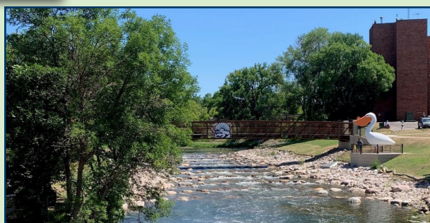
The deteriorating dam in Pelican Rapids, MN was modified into a Rock Arch Rapids winter 2022/2023. The ramp gradually steps down the water 5 feet over 12 arches.
