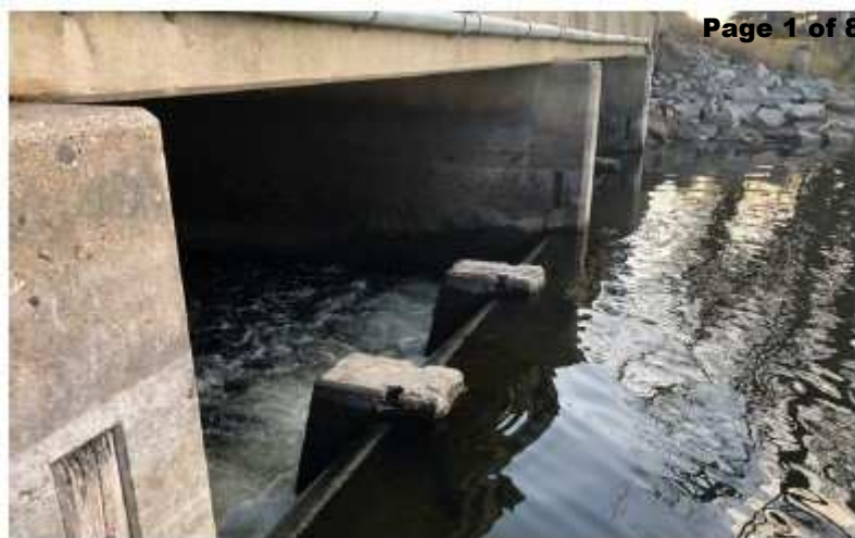
Control Structure at CR 108 Bridge 93
